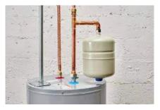
(sometimes called a thermal expansion tank) can help minimize the risk of pressure damage to the plumbing system. (This is normally not a problem on modern on-demand, tankless water heaters -- only tank-style heaters are subject to this problem.)
